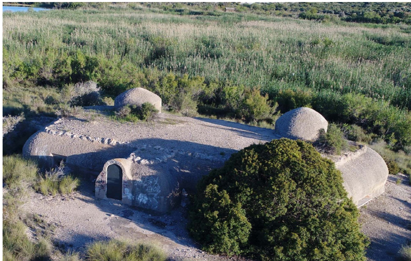
03. Bunker built between 1936 and 1939, developed on two levels in the centre of the Clot de Galvany lagoon, Spain. A. Martínez-Medina e P.J. Juan Gutiérrez, 2019
