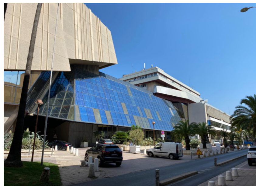
15. ACROPOLIS. The entrance hall (Agora) in the foreground. It is a single three-story open space for connecting the parts of the building and, if necessary, the two parts of the city "cut off" by the building. The 400-square-meter sunroof allowed natural internal ventilation and summer cooling in good weather. Photo credit: author, 2017
