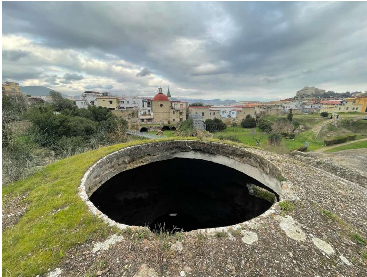
Pictures of the extrados of the dome of the so-called Temple of Mercury, detail of the oculus.
