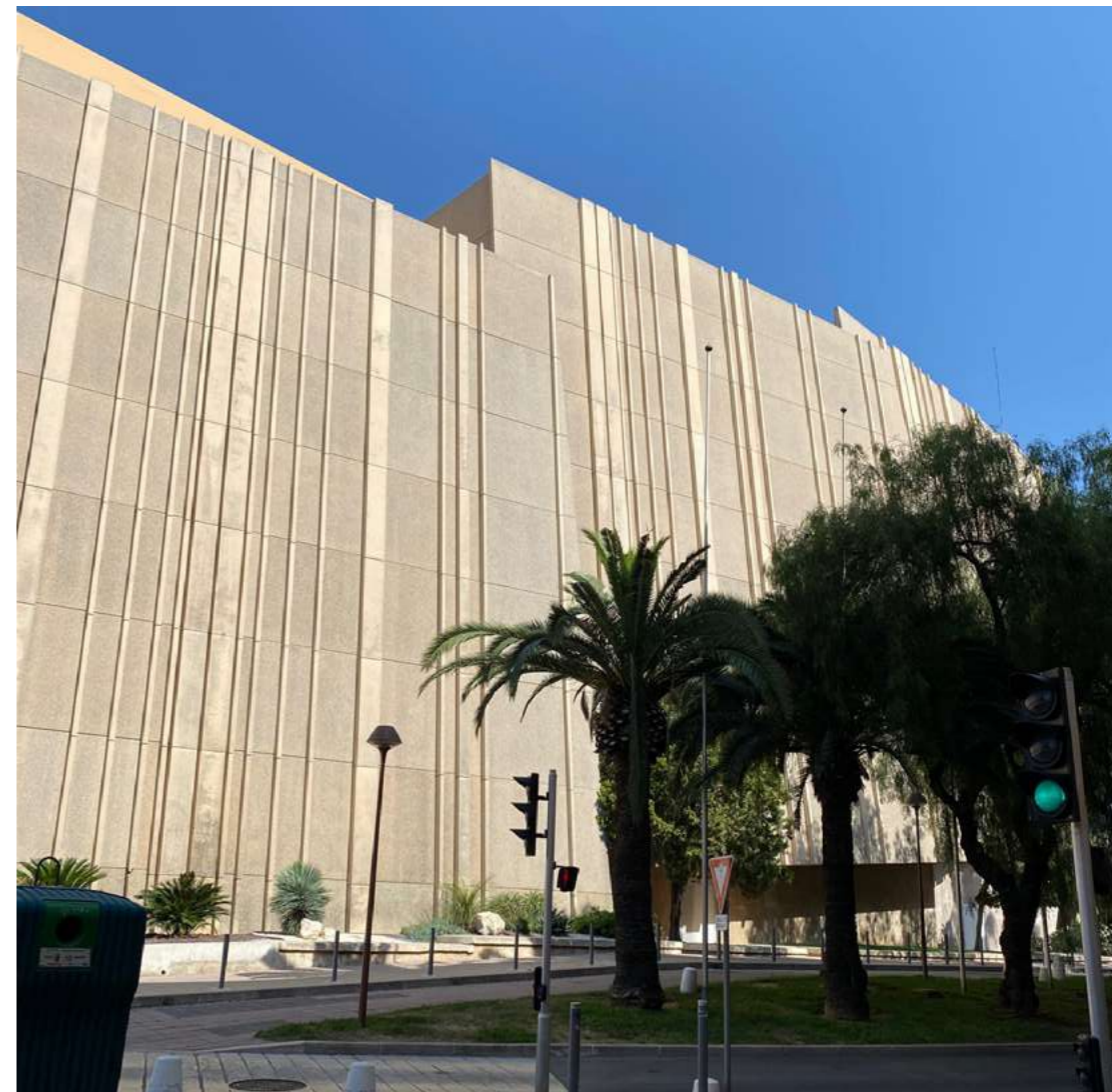
16. Detail of the exterior facades of the Auditorium. The precast reinforced concrete facades with irregular vertical reliefs were found to be articulately sloping inward toward the building, creating a sharp discontinuity from the surroundings. Photo credit: author, 2017
