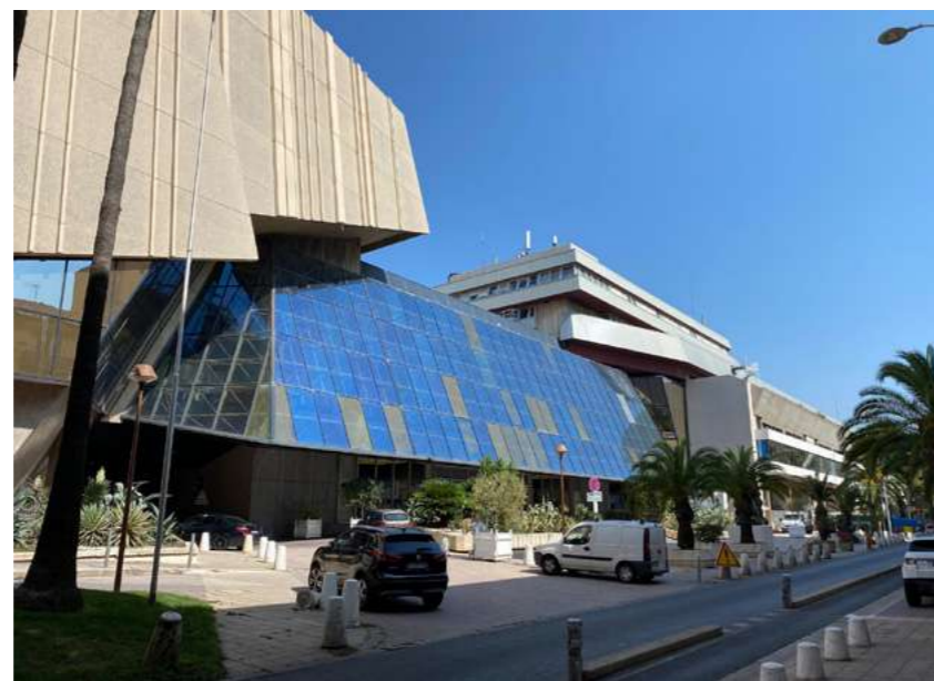
15. ACROPOLIS. The entrance hall (Agora) in the foreground. It is a single three-story open space for connecting the parts of the building and, if necessary, the two parts of the city "cut off" by the building. The 400-square-meter sunroof allowed natural internal ventilation and summer cooling in good weather. Photo credit: author, 2017
