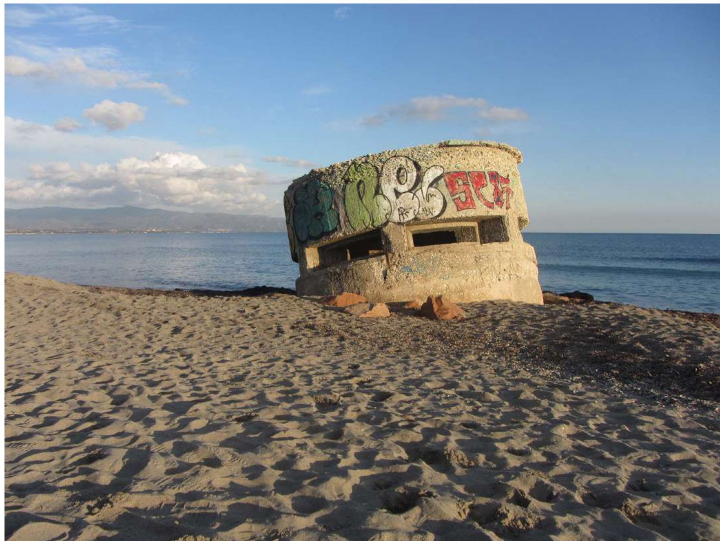
05. Bunker located along the coastline of Cagliari. Andrea Pirinu, 2018
