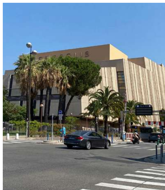
14. ACROPOLIS. The volume of the Auditorium for 2,500 people is highlighted. The 25 m construction module chosen for the entire project corresponds to the average length of the facades of the houses opposite the Multipurpose Center. Photo credit: author, 2017
