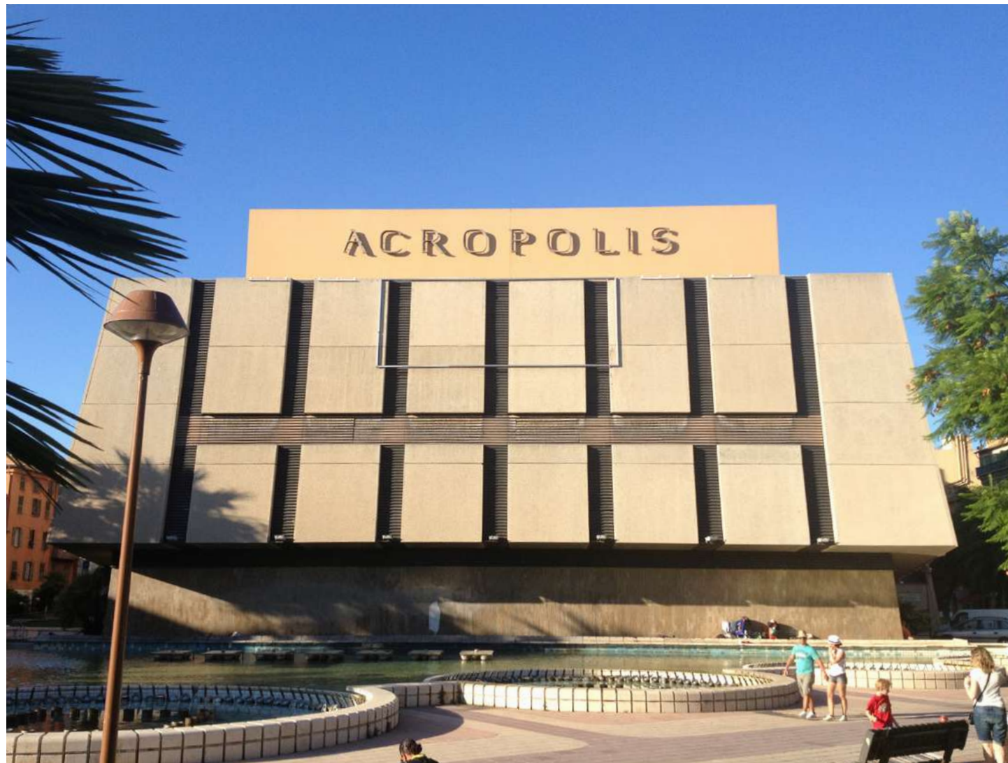
13. The southwest facade of the Multipurpose Center designed by G. Buzzi, P. Baptiste and P. Bernasconi (1981–1984) with consultancy on acoustic design by Prof. Eng. Lothar Cremer (formerly a consultant to Hans Scharoun for the Berlin Philharmonic) for the Auditorium. Photo credit: author, 2014
